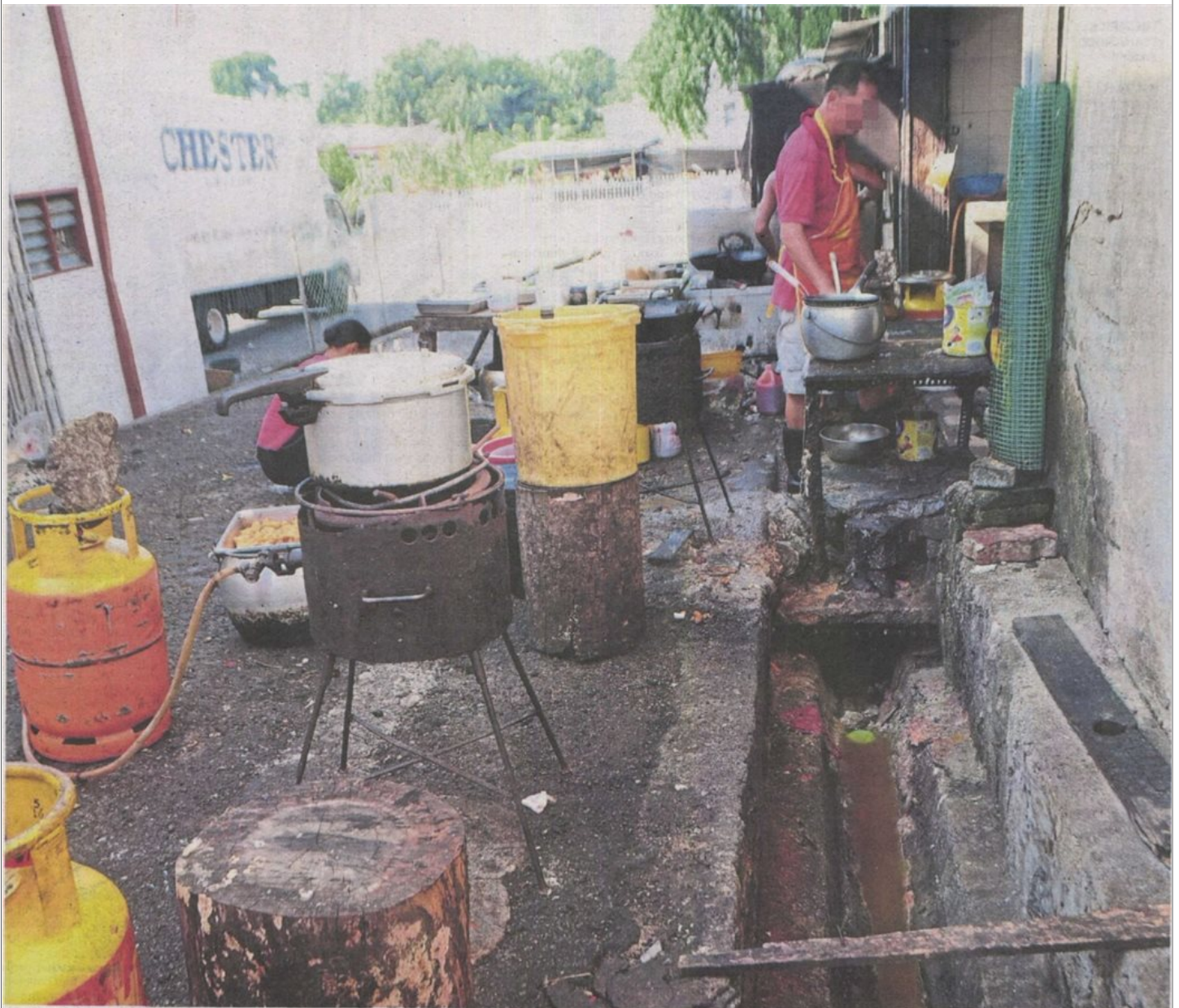
Breaking all the rules: The health department prohibits direct discharge of water from pipes into drains as well as washing plates or preparing food in back lanes. Only restaurants with fat, oil and grease (FOG) traps will be issued licences. This restaurant in Taman Megah, Cheras, however, is still operating as a result of poor enforcement. — GRACE CHEN/The Star
